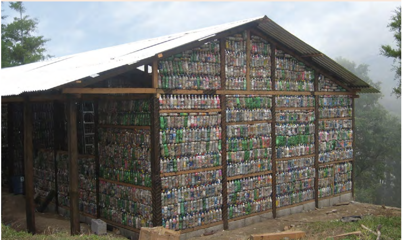
Example of a classroom built with ecobricks
